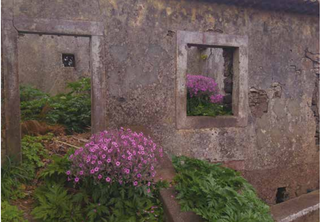
Fig. 16 Geranium maderense adorning an abandoned ruin at Ribeira de Vaca
