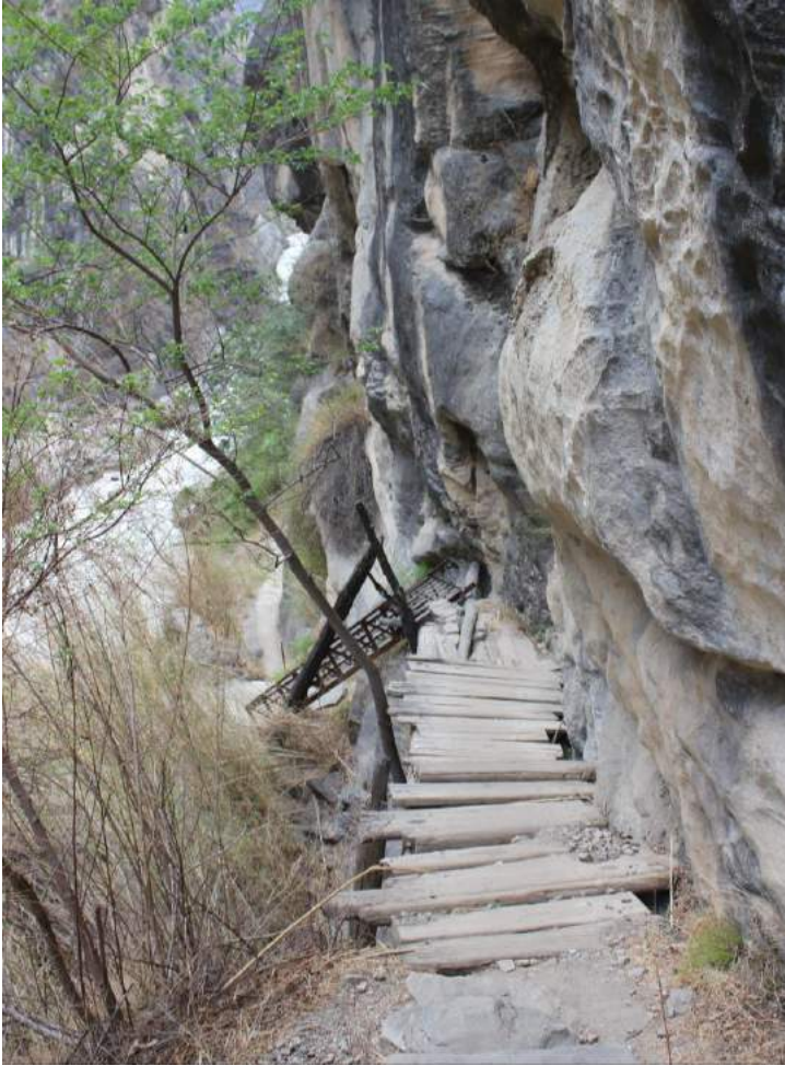
Figure 31 The steep and hazardous path down to the river.
