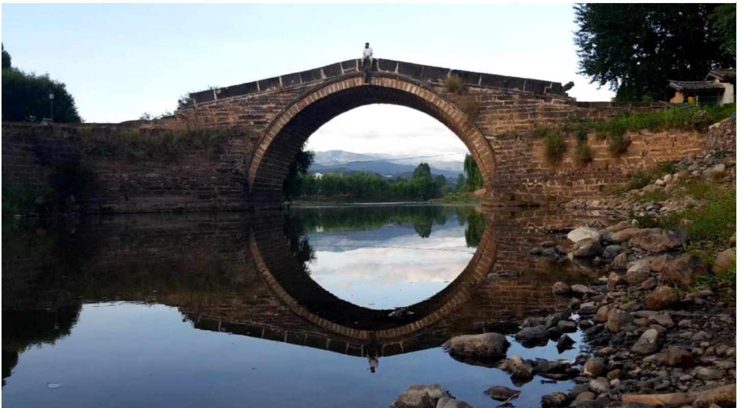
Figure 22 Yujin Bridge over the Heihui River, Shaxi.
